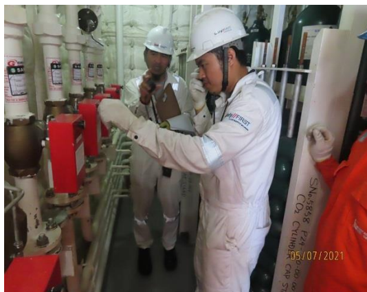
Preparation for Fixed CO2 System release in Cargo Hold
